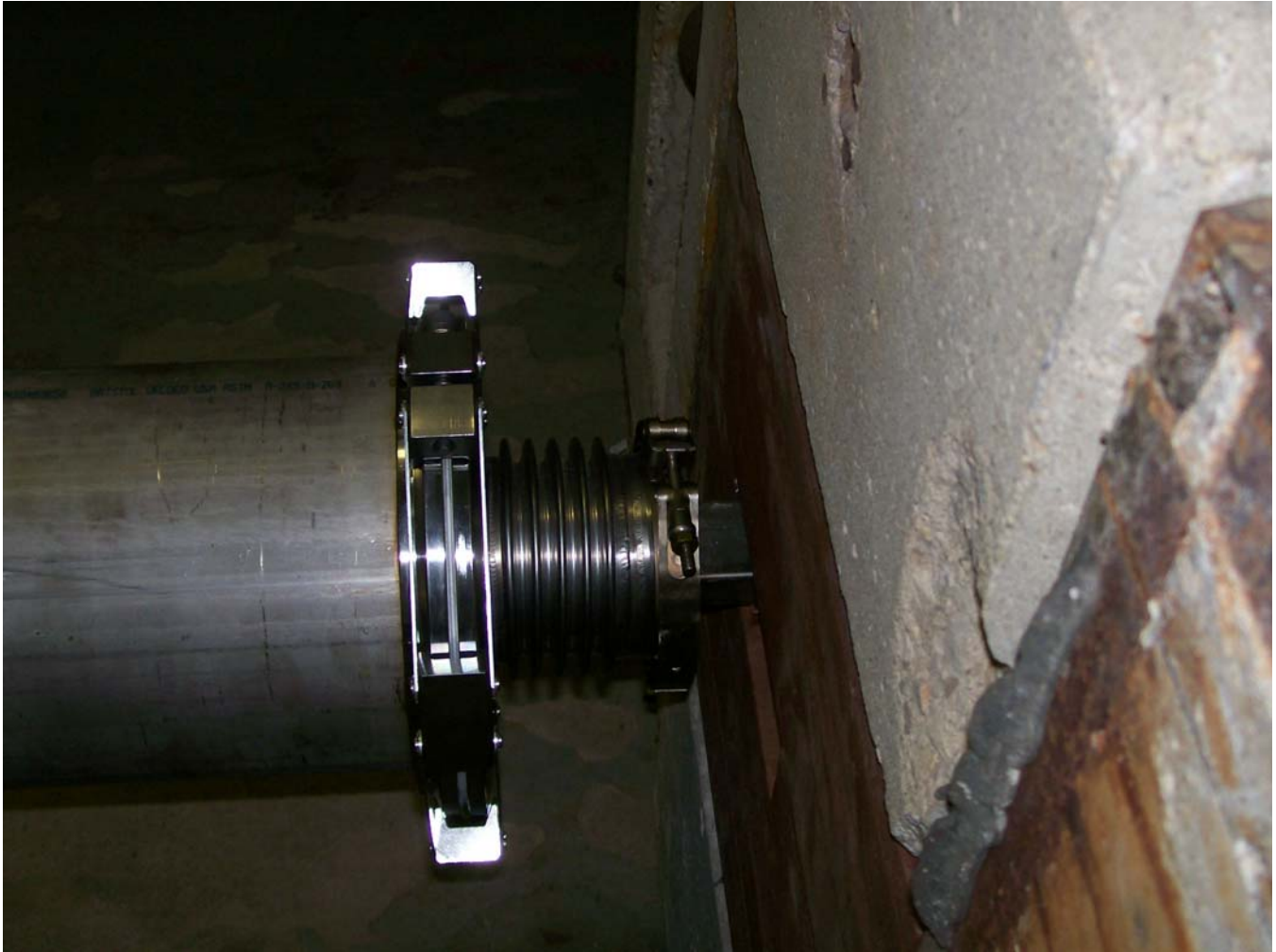
MTBABS UPSTREAM END
