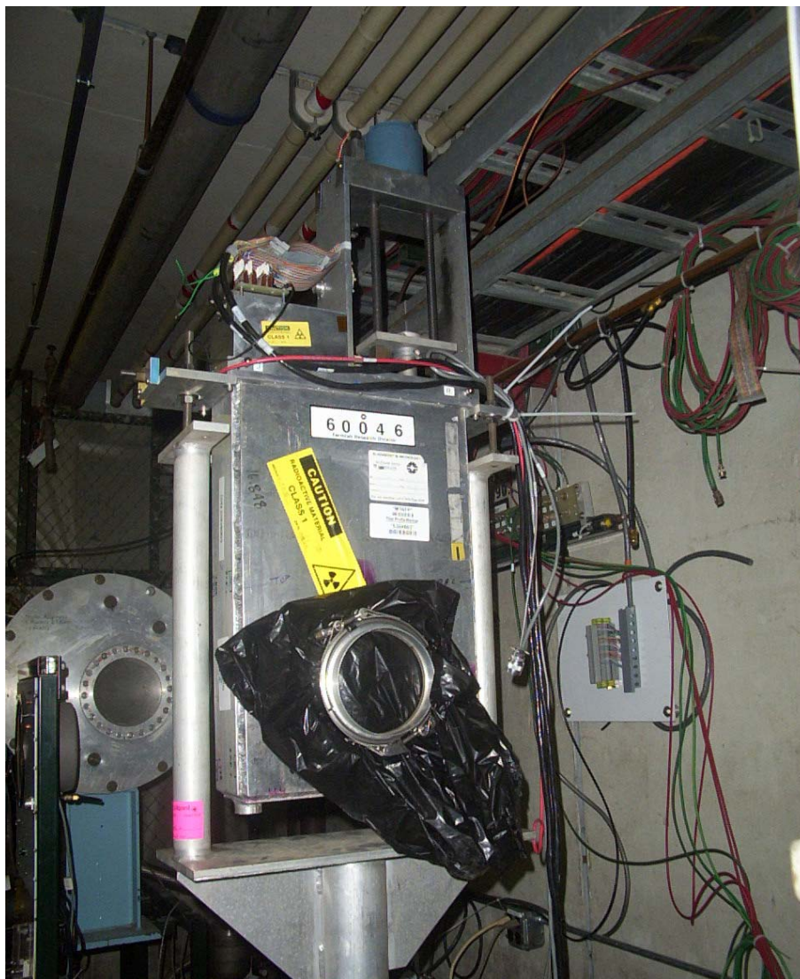
MT6FP Downstream (Looking Upstream)
