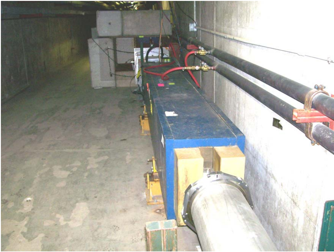
MT3U2 – LOOKING DOWNSTREAM
