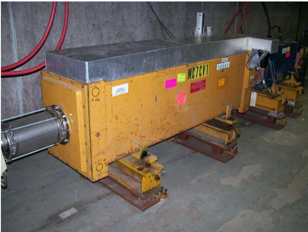
MT4CV1 UPSTREAM – BEAM RIGHT VIEW
