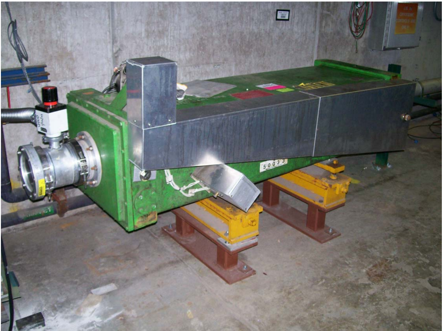
MT4CH1 UPSTREAM – BEAM RIGHT VIEW
