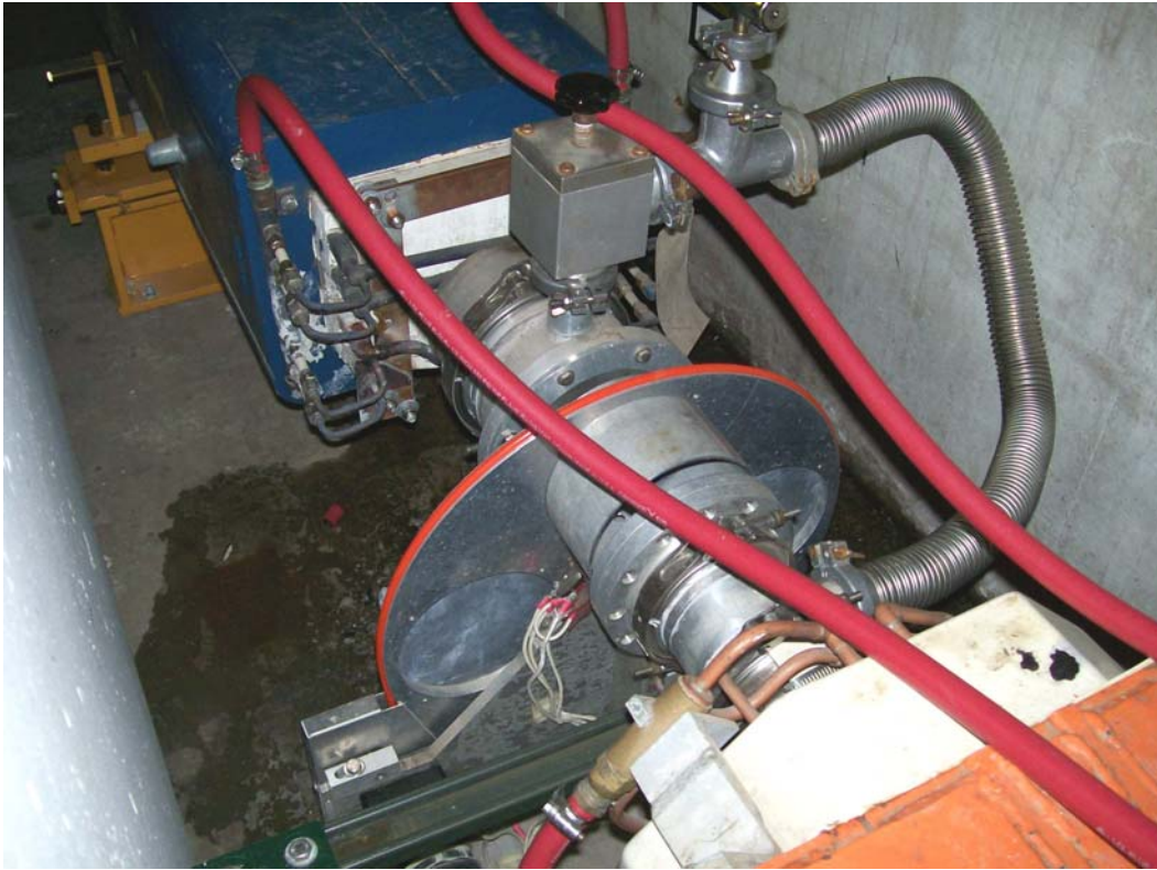
MT3CN2 LOOKING DOWNSTREAM
