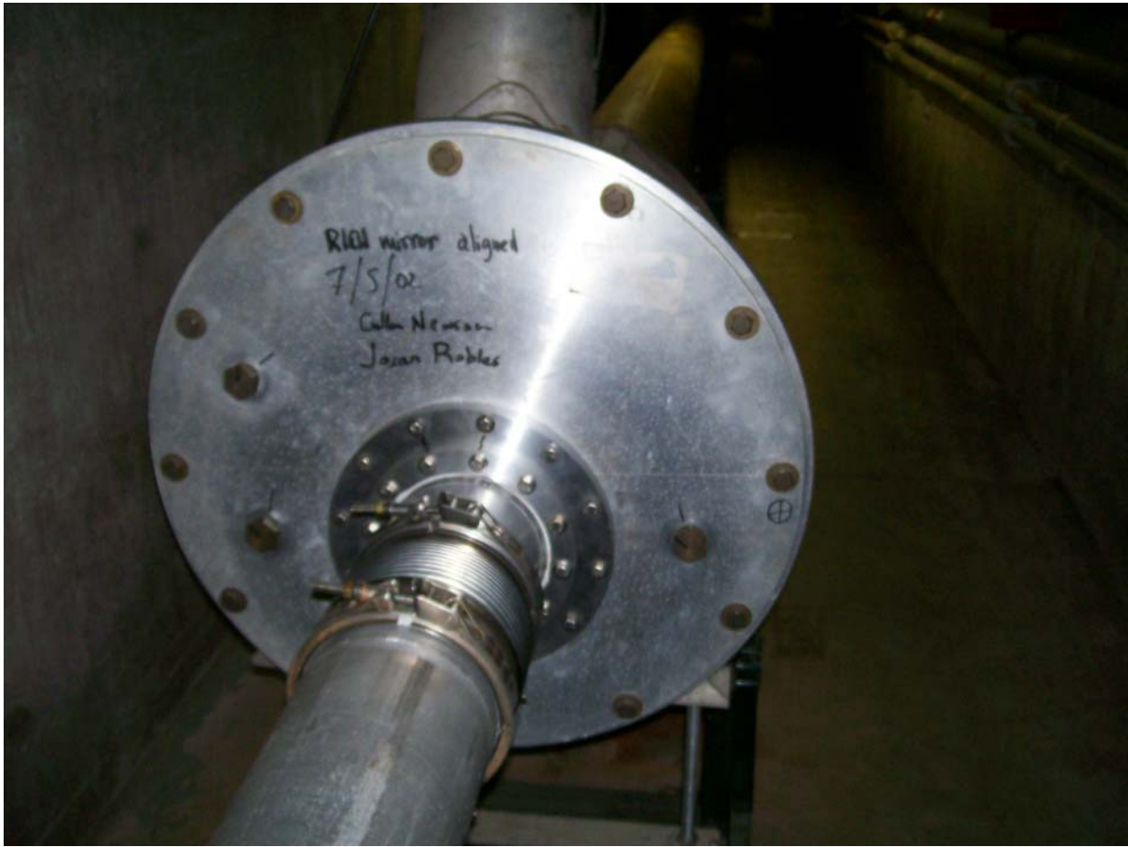
MT5CV1 DOWNSTREAM END (Looking Upstream)
