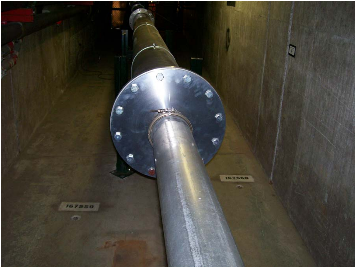
MT5CV2 UPSTREAM (Looking Downstream)
