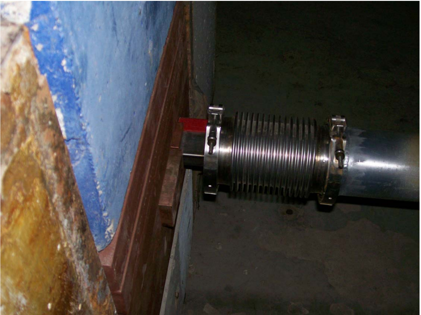
MTBABS DOWNSTREAM END (Looking towards Beam Left)
