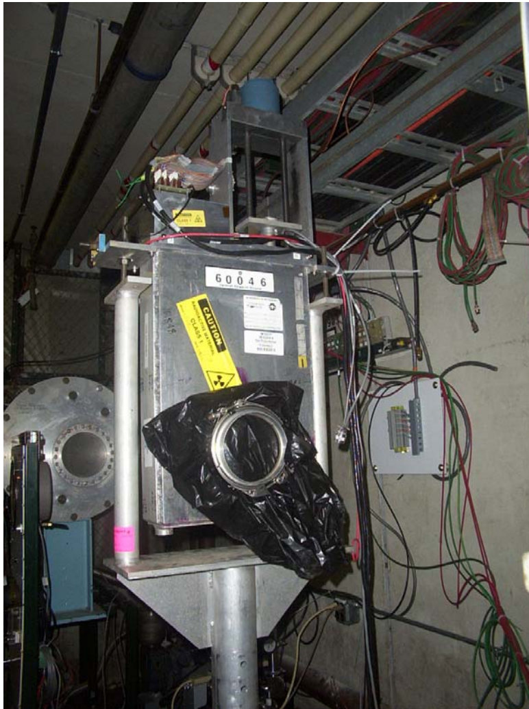
MT5CV2 DOWNSTREAM (Looking Upstream)
