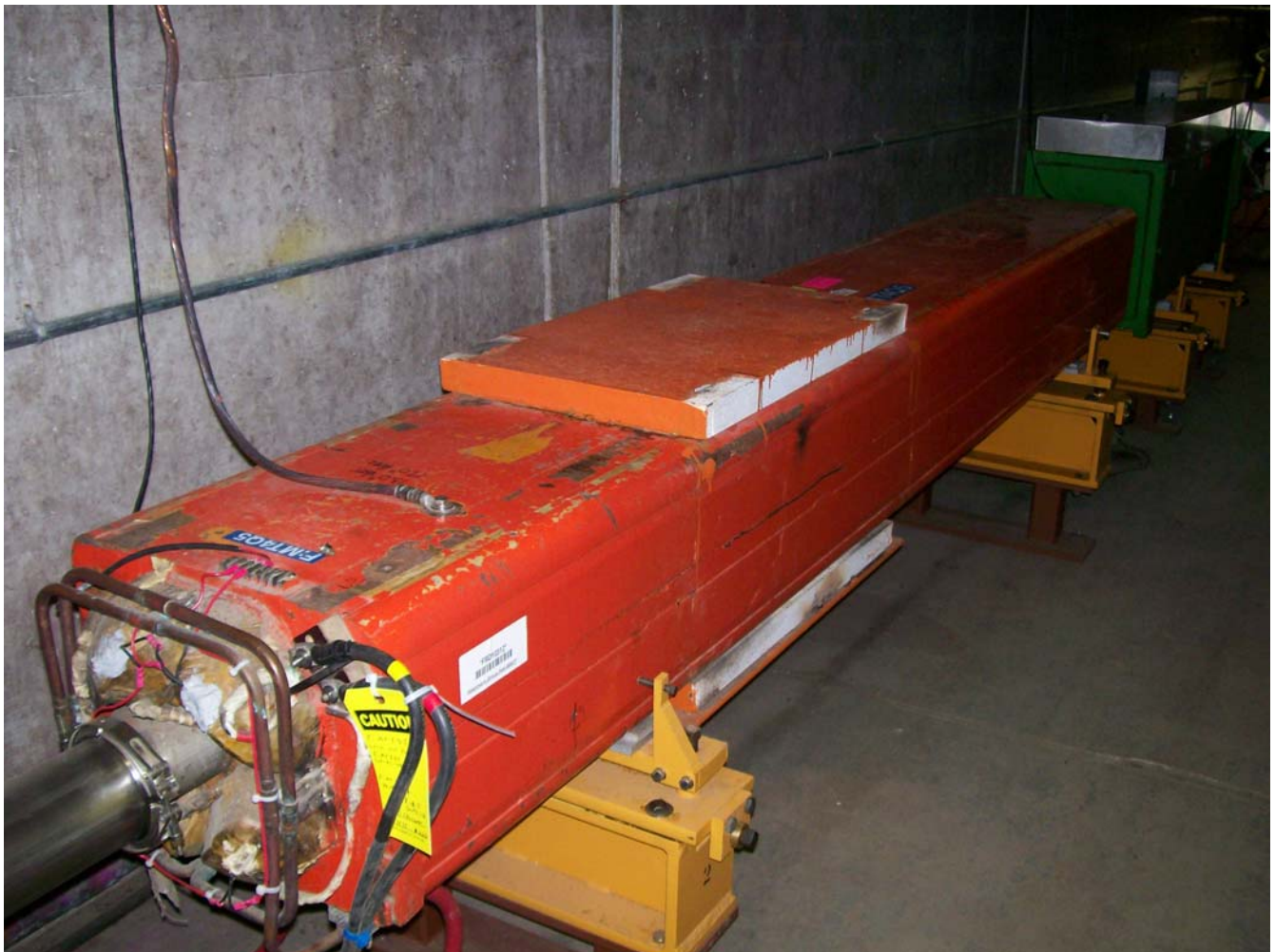
MT4Q5 UPSTREAM – BEAM RIGHT VIEW
