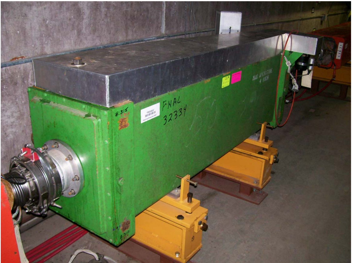
MT4CV2 UPSTREAM –BEAM RIGHT VIEW
