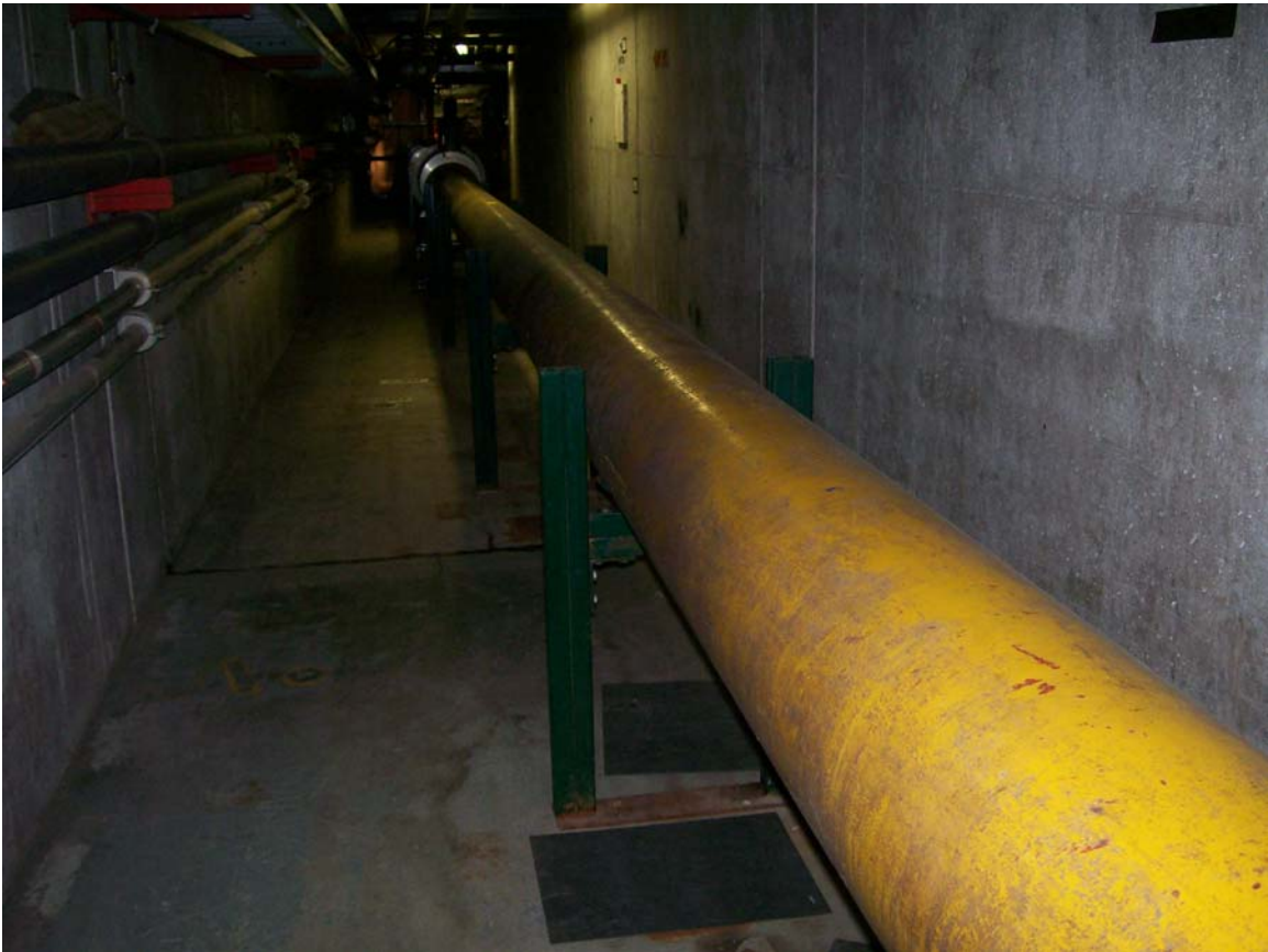
MT5CV1 UPSTREAM END (Looking Downstream)
