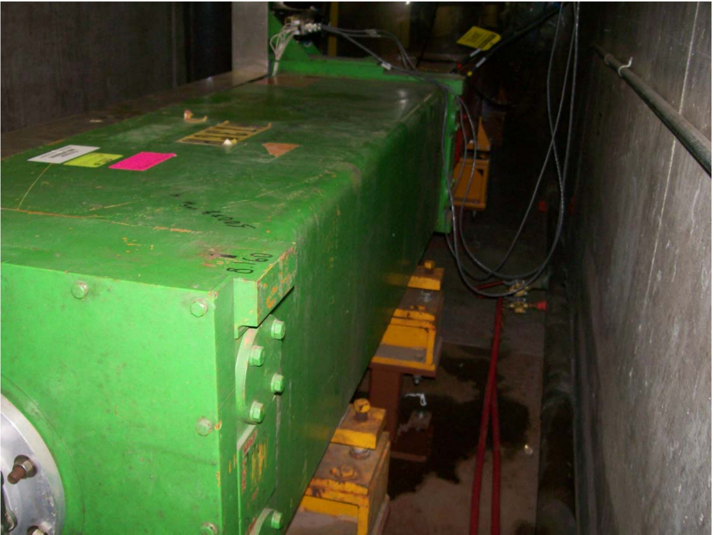
MT4CH2 DOWNSTREAM – BEAM LEFT VIEW (Looking Upstream)
