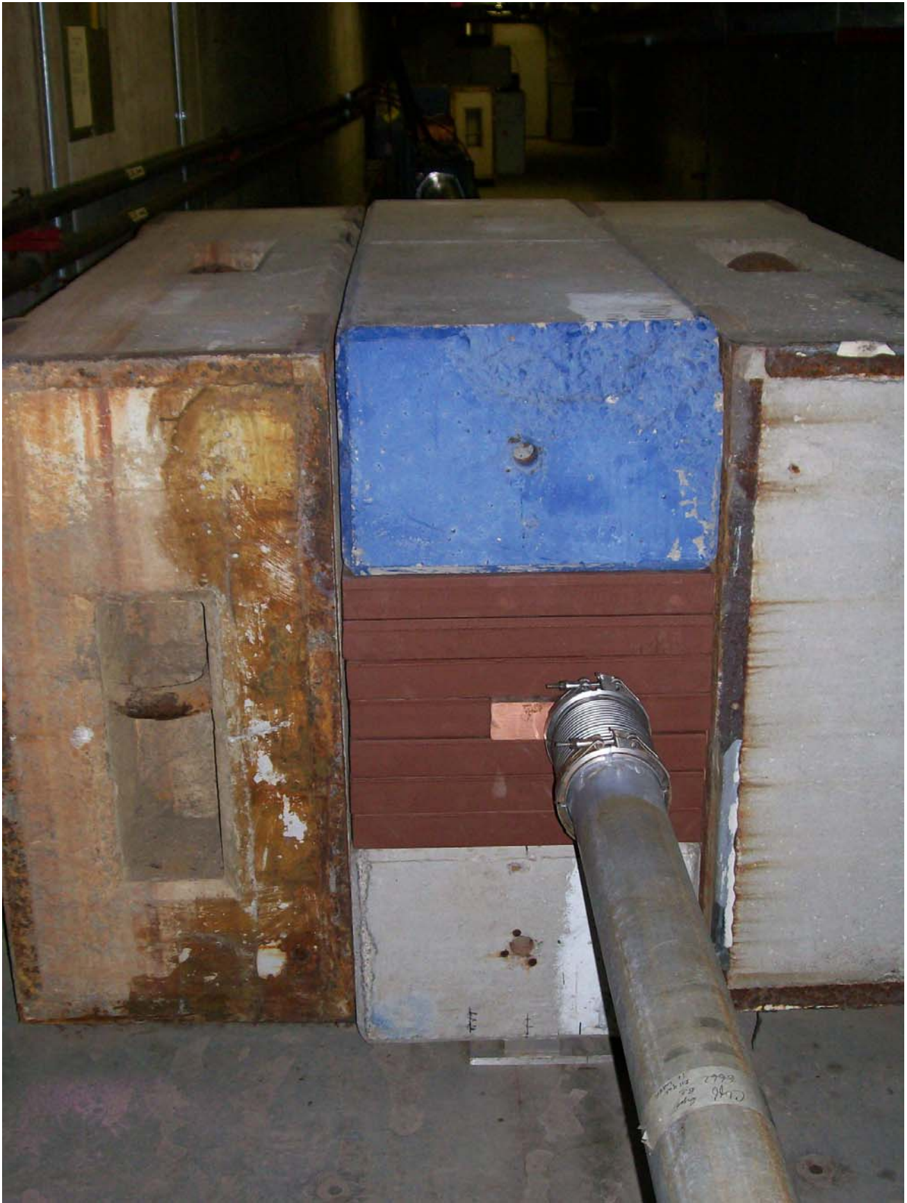
MTBABS DOWNSTREAM END (Looking Upstream)
