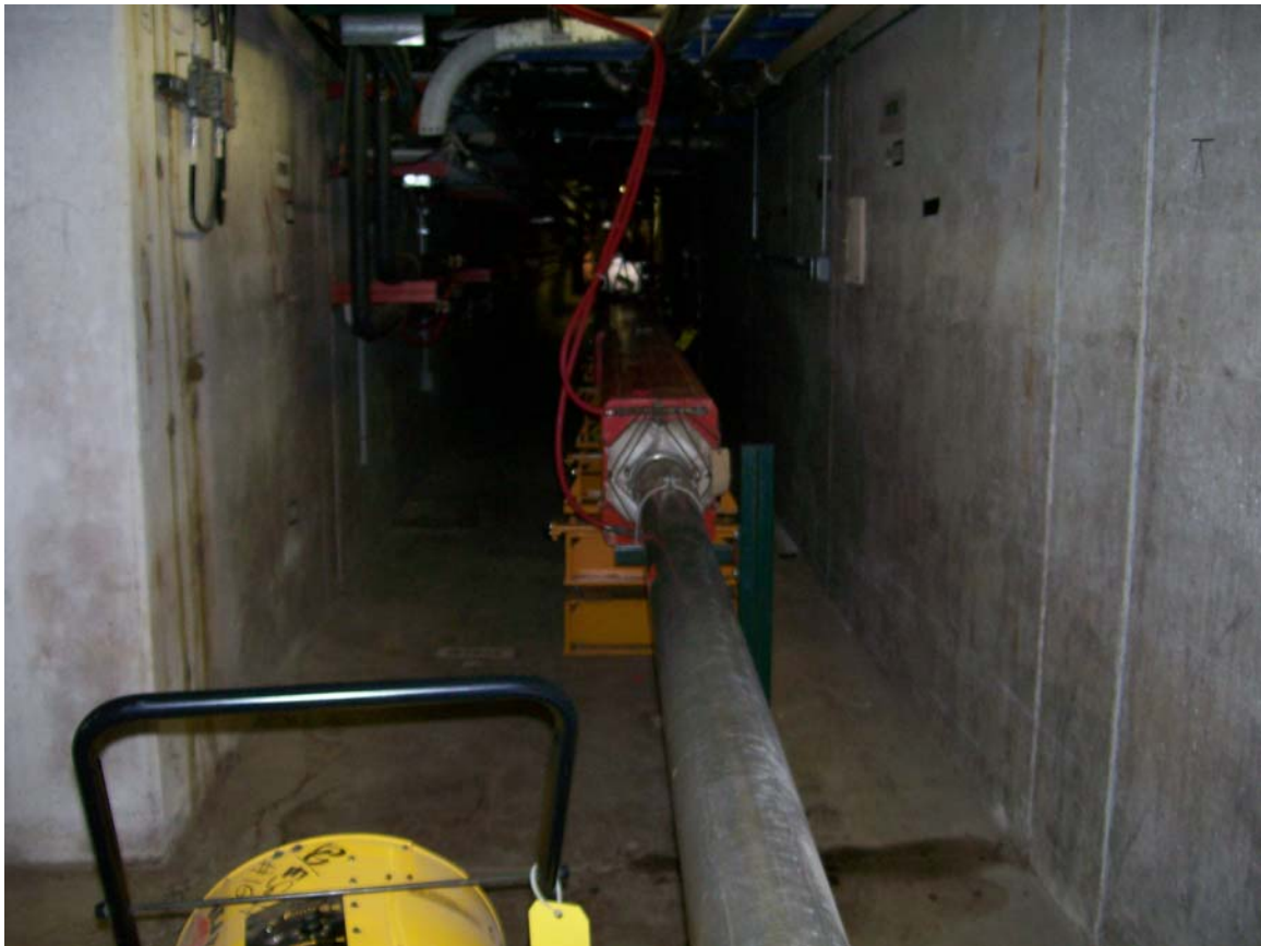
MT5Q1 UPSTREAM (LOOKING DOWNSTREAM)
