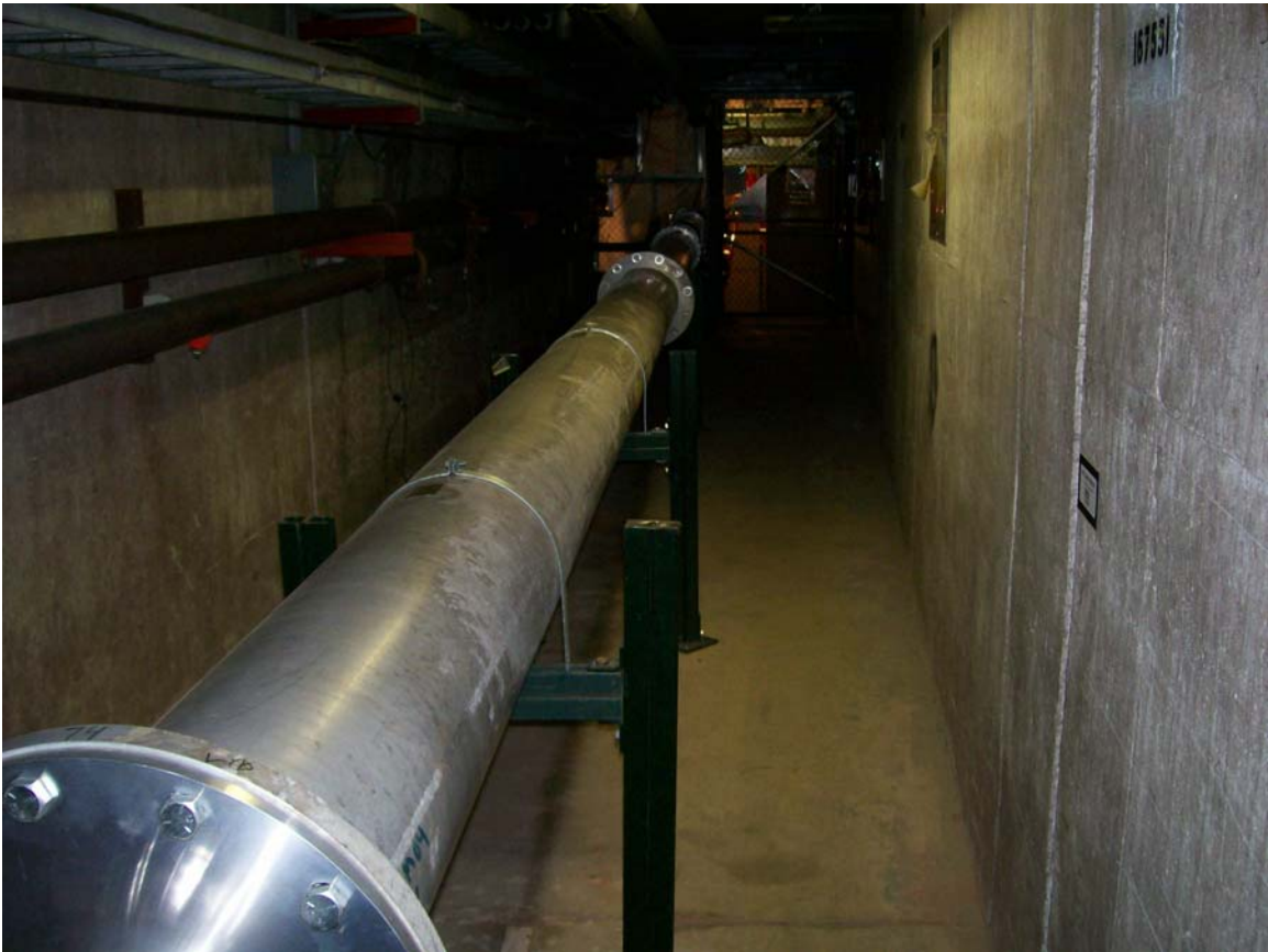
MT5CV2 UPSTREAM (Looking Downstream)
