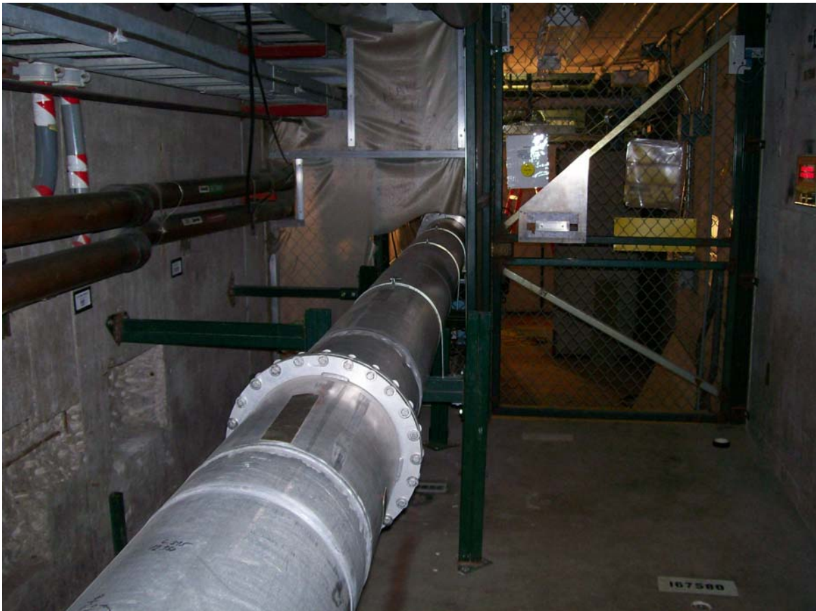
MT5CV2 (Looking Downstream)
